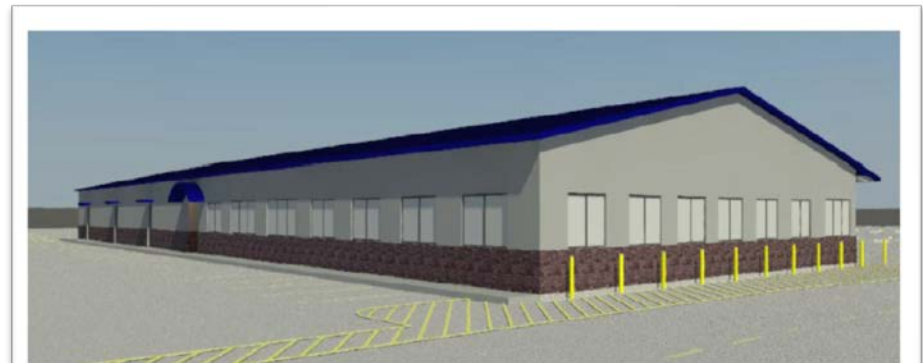
ADMIN./DISPATCH BUILDING, LOOKING SOUTHWEST
